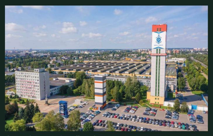
One of the city's tallest landmarks is the 84-meter tower of the Mogilevliftmash testing facility. From the top, all of Mogilev and its surroundings can literally be seen at a glance. The building contains eight open-through shafts used for trial runs of experimental units and components, as well as test drives of serial elevators before they go into production. This tower welcomes employees and visitors from afar as they approach the plant.
